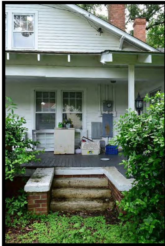
Figure 8: Whitley House, Looking Southwest.
