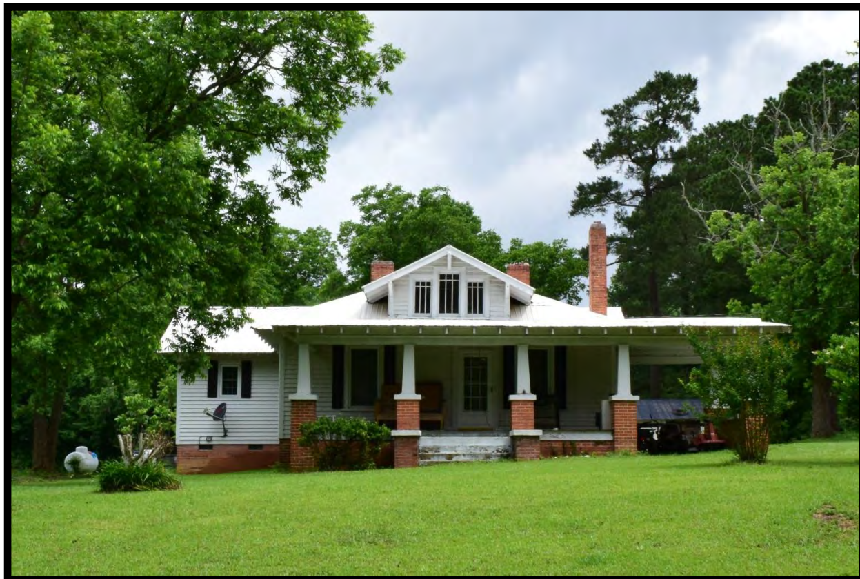
Figure 17: 3838 Black Creek Road, Looking North.
